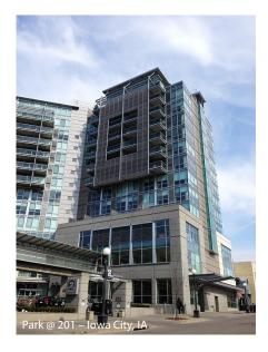
Ask for balcony doors that are side-stacking with window wall systems, for matching runs of framing and accessories, single source responsibility, one warranty, one finisher, one set of shop drawings and calculations **Review:**
